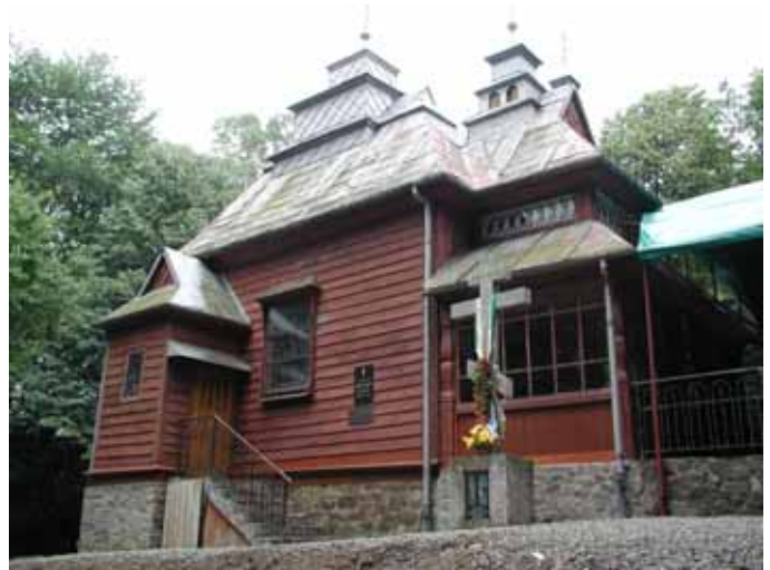
Picture 25. The chapel on Sycamore Hill near Wysowa.
